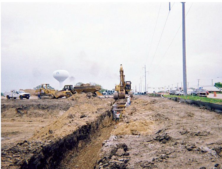
The replacement PVC pipe was laid in a new alignment.
