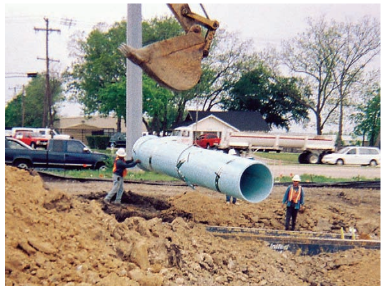
DR25, AWWA C905 PVC pipe was specified as the replacement pipe because it was readily available.
