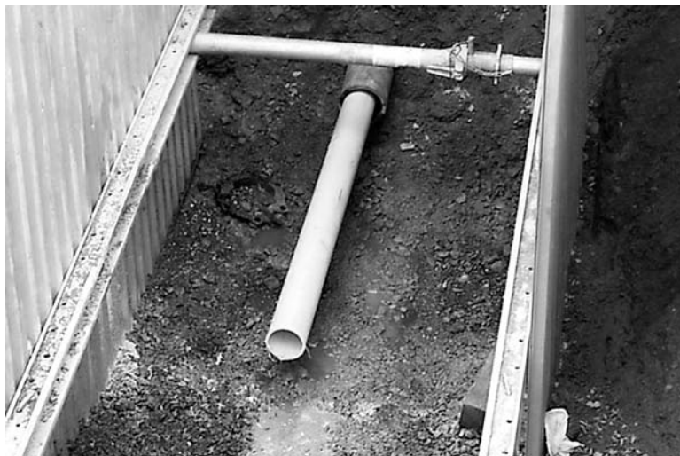
Fig. 13.14 Starting stock inserted into host pipe.
