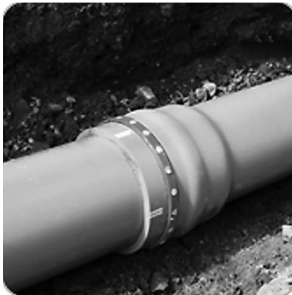
Fig. 13.2 Pin-and groove gasketed joint.
