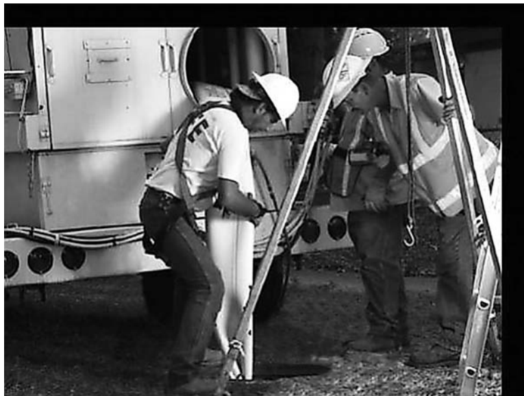
Fig. 13.17 Heated liner being winched into a manhole.
