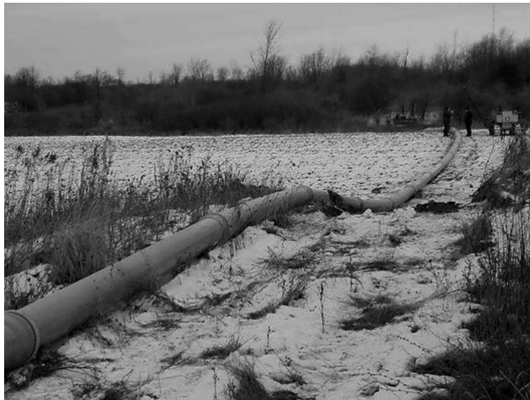
Fig. 13.8 Preassembled PVC pipes.
