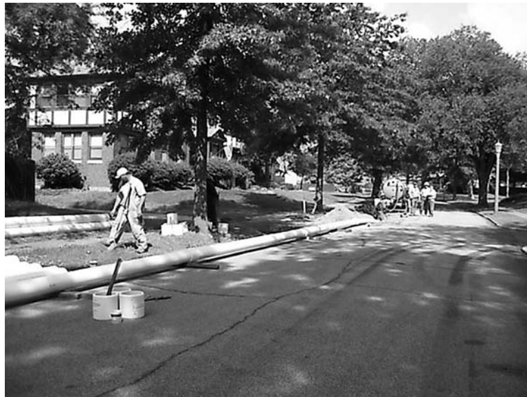
Fig. 13.10 Pipe string during pullback operation.
